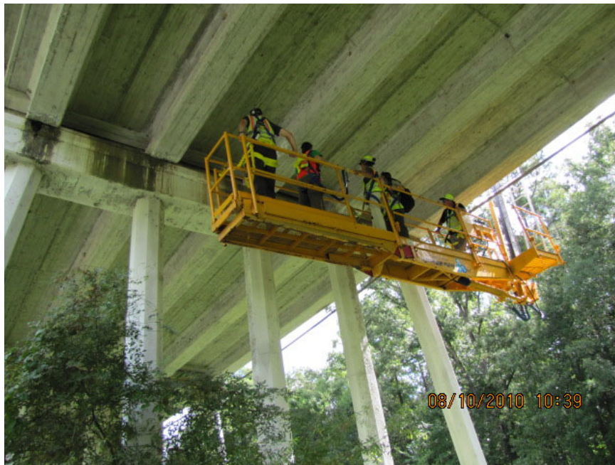
Figure 14. Biologists use a snooper truck to assess expansion joints and concrete caps over deep water (photo provided by Georgia Department of Transportation).
